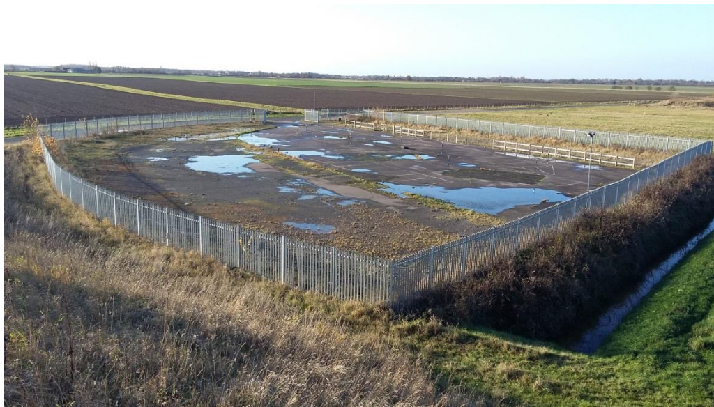
Figure 1: The Site at present
